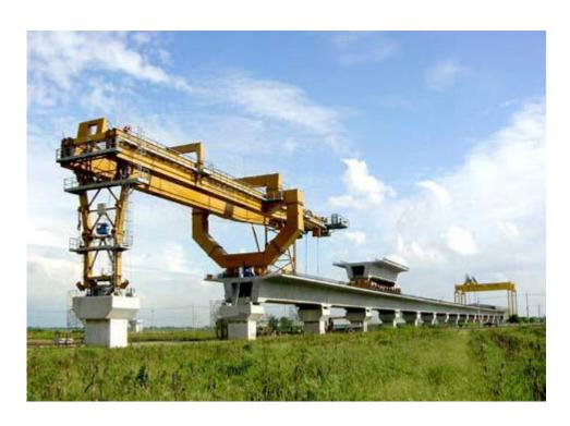
Client: HBP Supplied equipment: Launching gantry, tyre trolley portal crane Capacity 915 t
